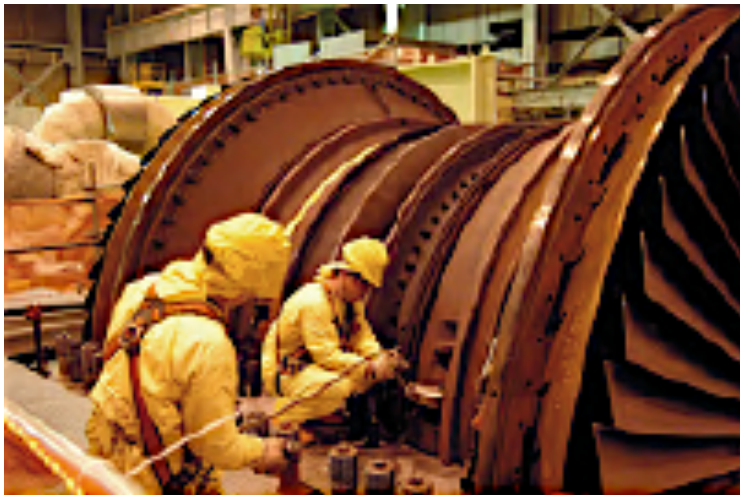
LOW PRESSURE- BLADE RINGS (82Bolts)
